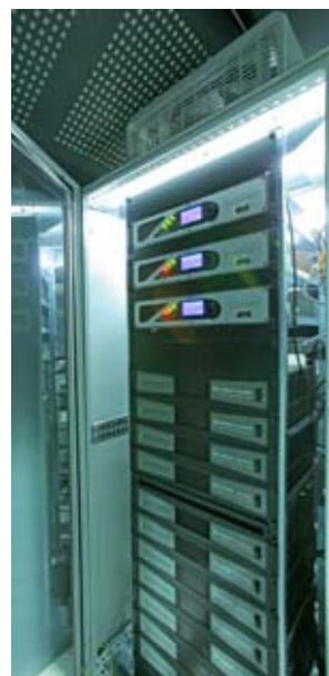
The heart of an MCR system. 19" racks with sound processors and amplifiers.
